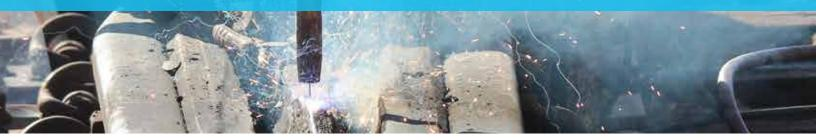
**Railroads report that traditional repairs to frogs and diamond inserts often only last weeks to a few months before requiring additional maintenance.** These specialty track components are manufactured out of cast austenitic high manganese steel known for its excellent work hardening characteristics and high toughness. However, this material creates a unique challenge to repair or refurbish in the field as it cannot exceed 500 degrees Fahrenheit.
